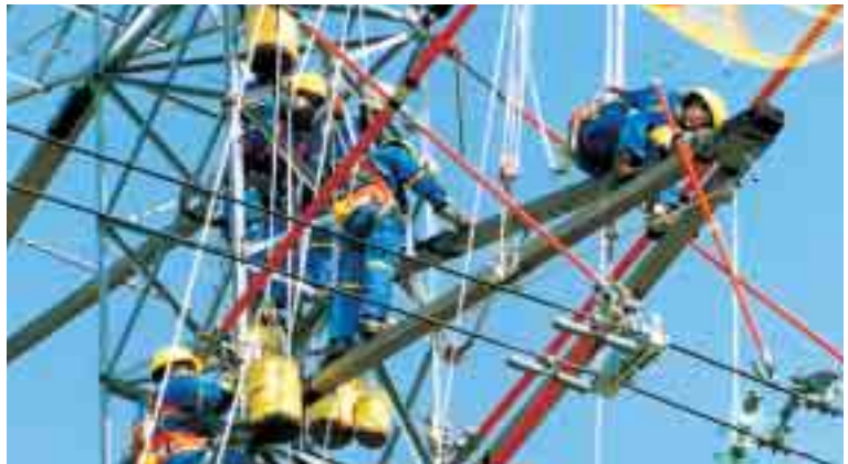
Live-line maintenance work in progress.
