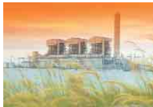
A scenic view of Manjung Power Plant.
