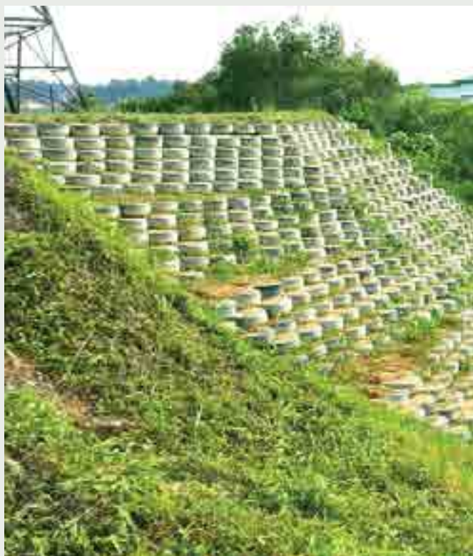
Protected slope using used tyres
