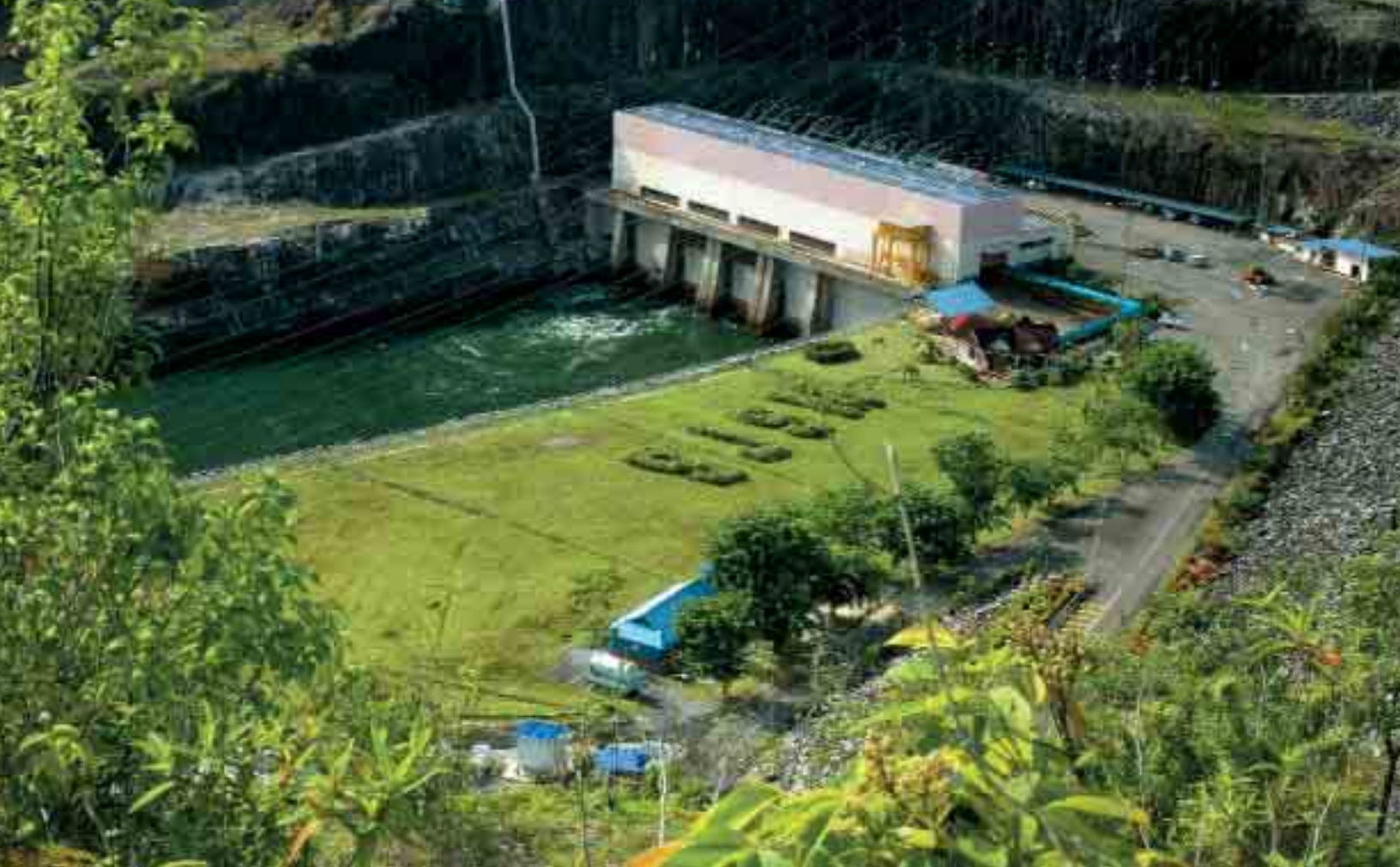
A view of Kenyir Power Station in synergy with nature.
