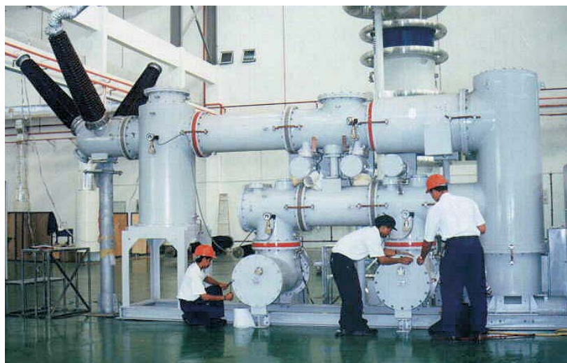
Maintenance and inspection works of GIS at TSG in progress
