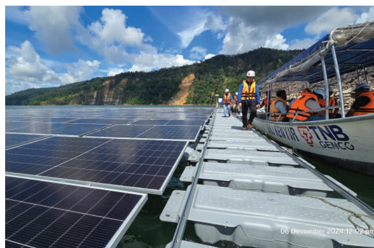
➡ Pilot Floating Solar PV located on Kenyir dam with a capacity of 100kWac.
