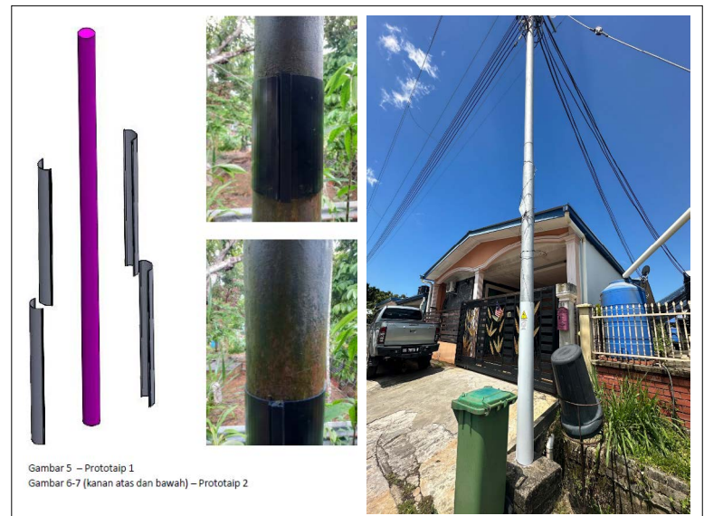
Installation of pole covers to prevent human and livestock contact with steel poles, reducing the risk of electrocution.
