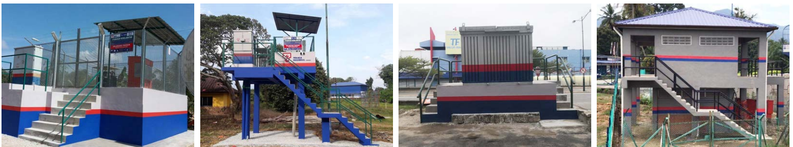
Flood proofing measures are implemented to reduce asset exposure, minimise service disruption and support faster restoration following flood events.
