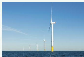
Blyth Offshore Windfarm
