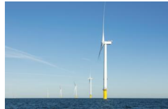
Blyth Offshore Windfarm
