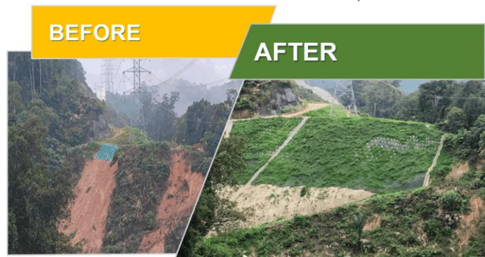
Figure 6.18: Transmission Tower Foundation Before and After the Implementation of Soil Nailing with Steel Grid Netting
