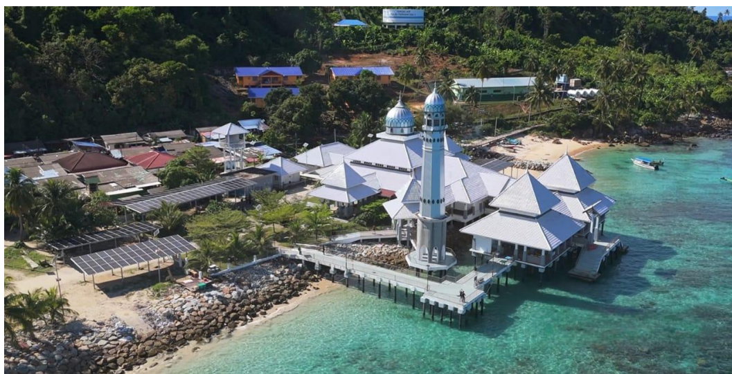
Figure 7.5: Solar BIPV system at Masjid Pulau Perhentian (118.8 kWp)
