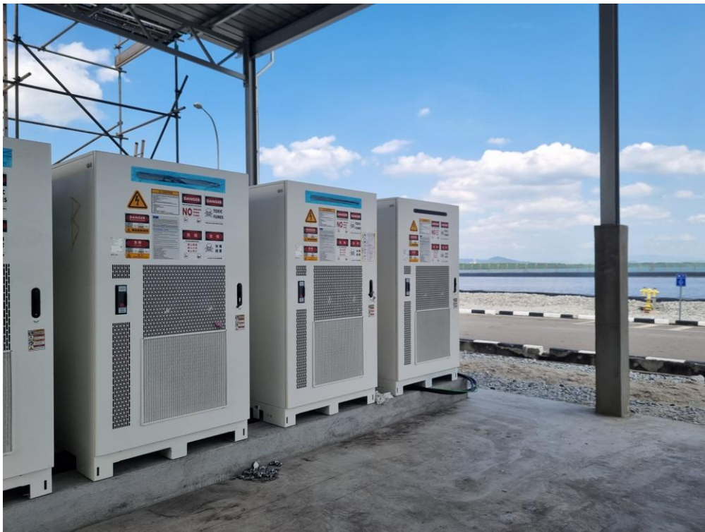
Figure 7.11: Installation of 1 MWh BESS under Project REACH
