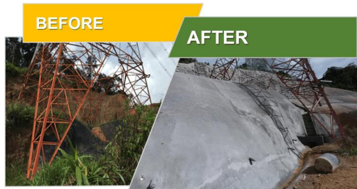
Figure 6.17: Transmission tower foundation before and after the implementation of soil nailing with gunite.
