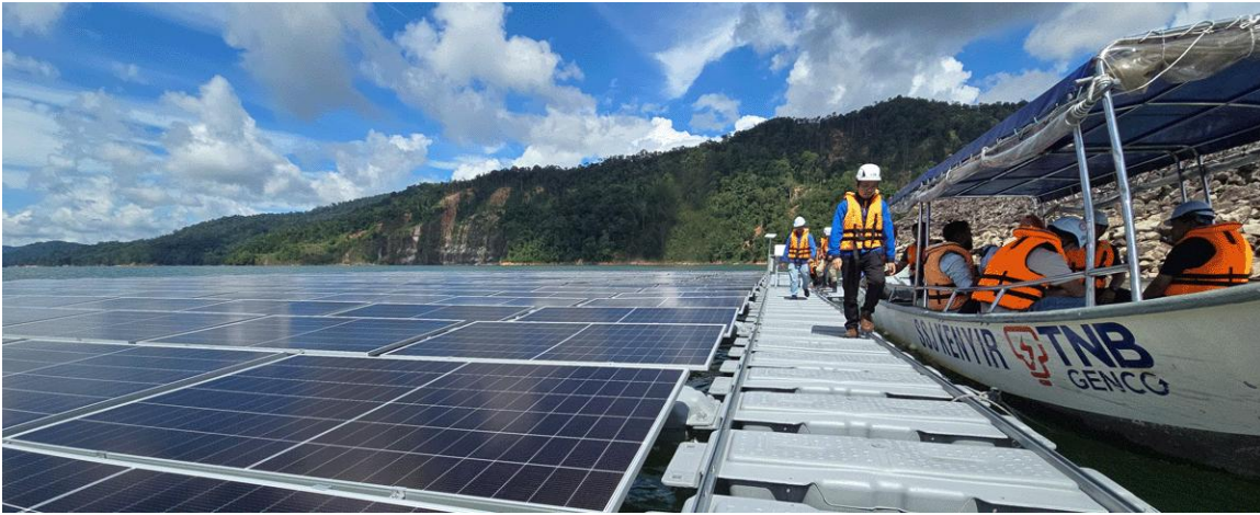
Figure 7.8: Floating solar pilot project at Stesen Janaelektrik Sultan Mahmud, Kenyir Dam
