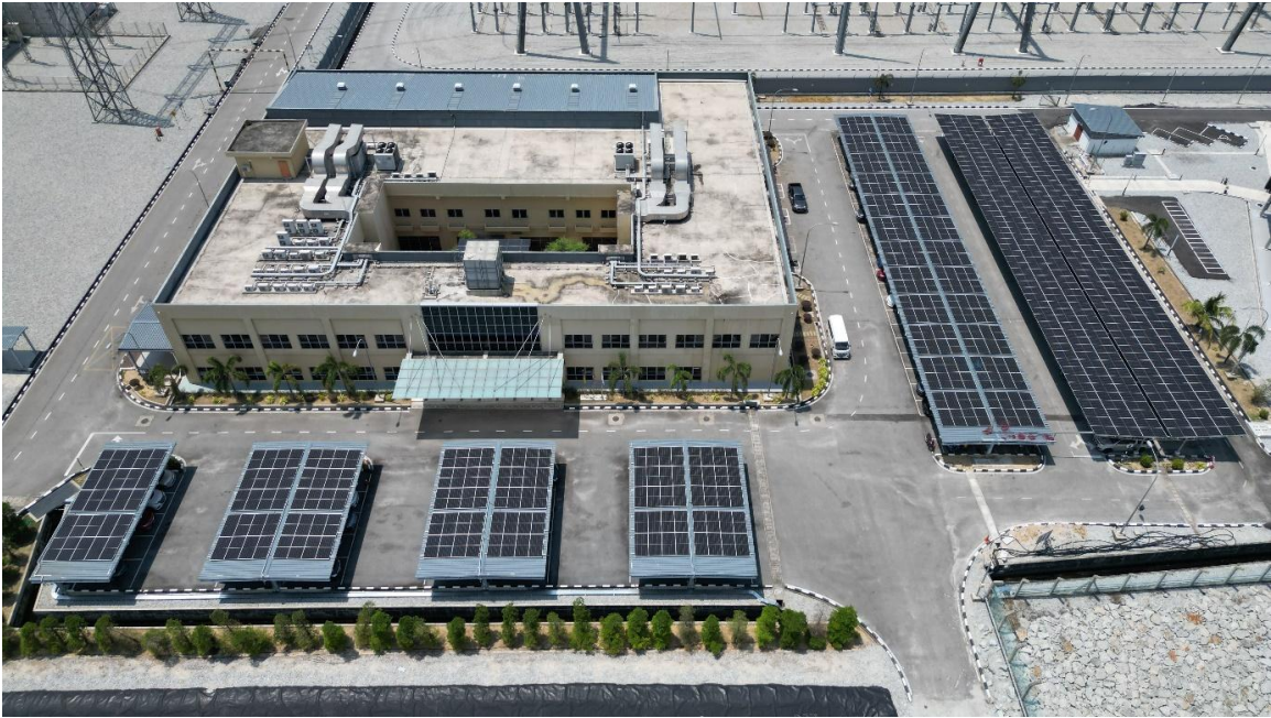
Figure 7.10: Installation of 500 kWp rooftop solar PV under Project REACH
