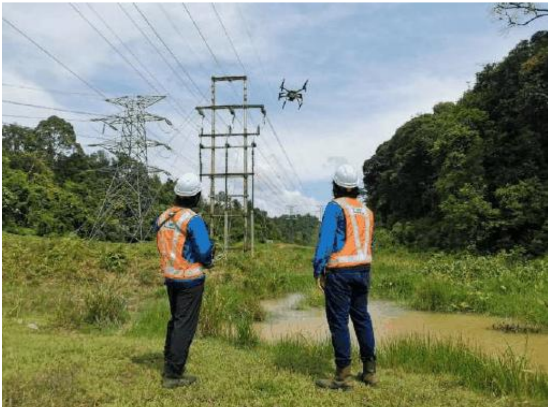
Figure 3.9: UAS application in MV overhead line inspection and maintenance regime.
