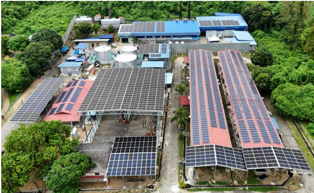
Figure 7.6: Solar PV installation at Pulau Tioman
