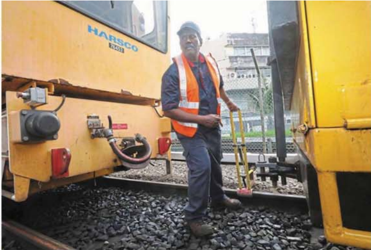
Iruthayaraj using an earthing device during maintenance work on a railway track.
