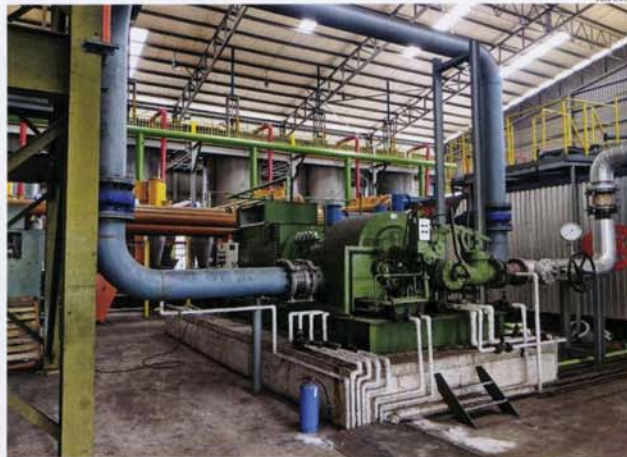
The group's REEP in Telok Gong, Klang, is expected to commence operations by year-end
