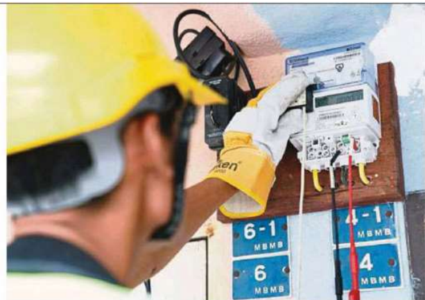
A smart meter being installed by a TNB worker in Melaka.
