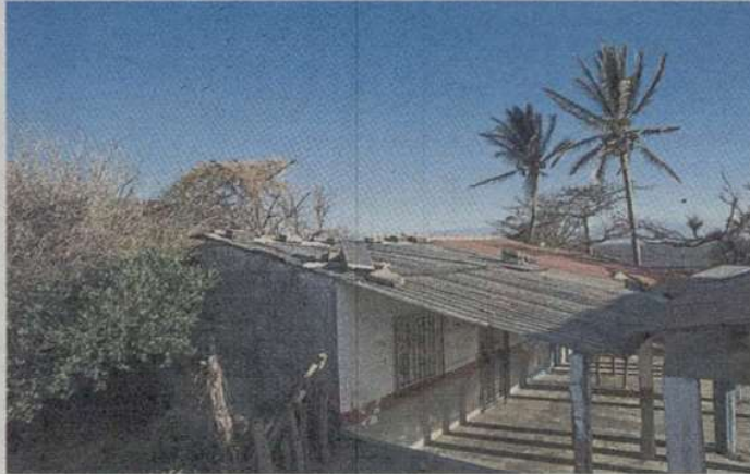
A solar panel, instaled by Guerra, is seen on a building in Cachimbo
