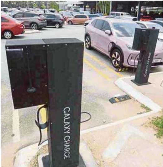
A distributed grid of homes with solar panels, batteries and EVs could turn households into both consumers and suppliers of electricity.
