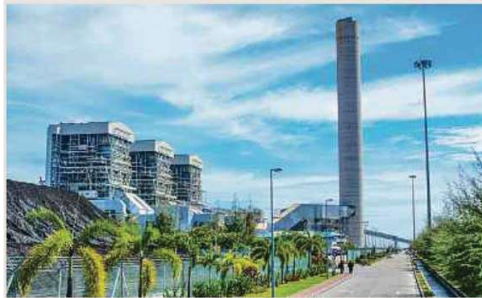
The students visited the Sultan Azlan Shah Power Plant in Manjung, which exposed them to the operations of the power station.
