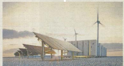
Hasilwan made history to power an entire highway operation under the Net Energy Metering scheme
