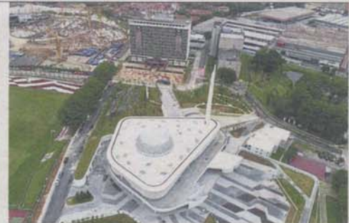
An overview of the complex. While traditional mosque elements are retained, the design also caters to the changing times and needs of the people.
