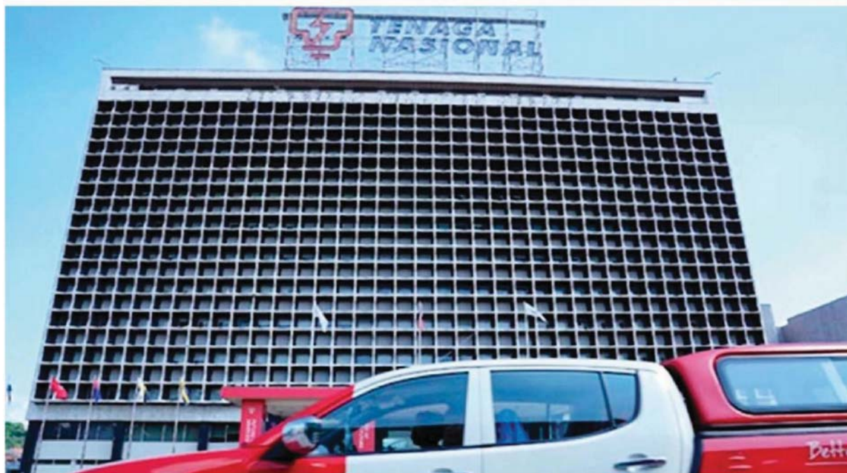
Tenaga guides for electricity demand growth of 2.5 to three per cent in 2024, driven by additional demand from new data centres. — Bernama photo
