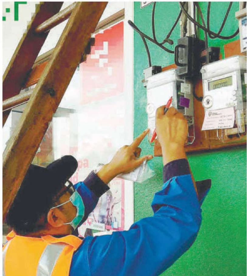
Smart meters automatically record electricity usage and transmit data to TNB via radio frequencies for real-time monitoring and billing, while identifying tampering cases. – PIC COURTESY OF TNB
