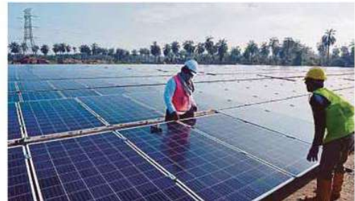
Tenaga Nasional Bhd's first large-scale solar project in Kuala Langat, Selangor, has a generation capacity of 50MW with DC install capacity of 78MWp.
