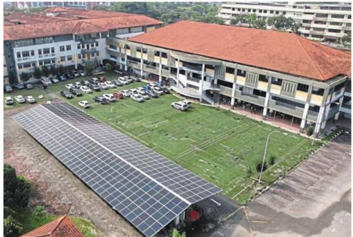
Aerial view of the solar panel array sheltering a carpark at SJK(C) Kuo Kuang 2. — Courtesy of SJK(C) Kuo Kuang 2.
