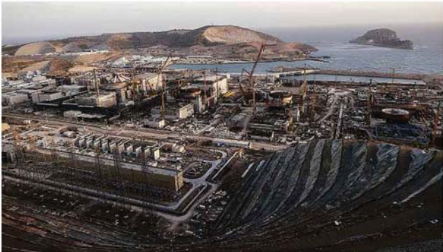
Turkiye is building the Akkuyu nuclear powered plant. AFP PIC
