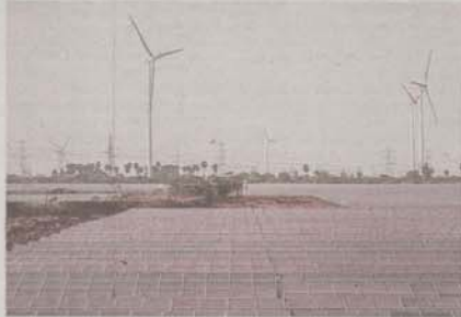
Researchers and industry players say expanding RE capacity will require corresponding improvements to the electricity grid
