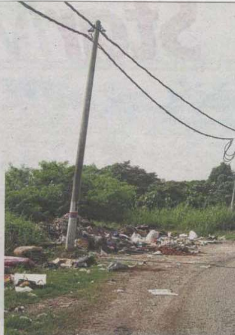
The burning of rubbish by unscrupulous parties on the roadside of Jalan Kebun Nenas in Klang had damaged the TNB cables above.
