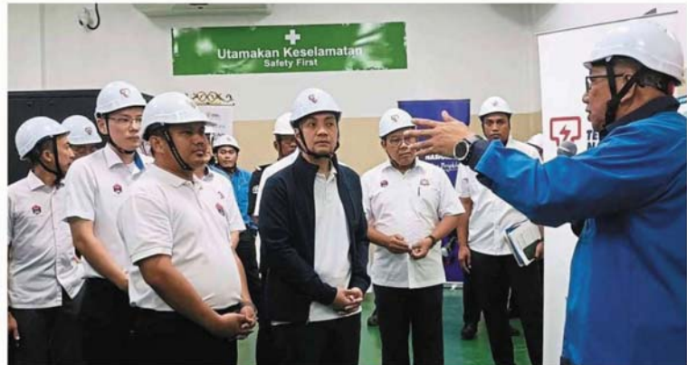
All ears: Onn Hafiz (centre) listening to a briefing from Tenaga Nasional Berhad during his visit to the Kota Masai Main Intake Substation in Pasir Gudang, Johor Baru.
