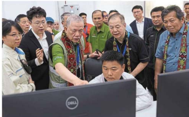
Promising alternative: Fadillah (third from left) visiting the Batang Ai Solar Control Room in conjunction with the Petra Squad Sarawak zone programme near Sri Aman. — Bernama
