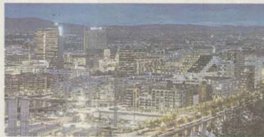
In Oslo, Hafslund Oslo Celsio is tapping into a main sewage pipe to provide heat and hot water for 13,000 apartments
