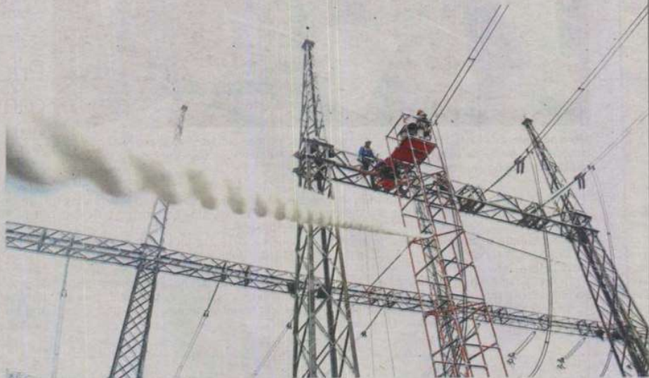
Enough supply: TNB maintenance personnel work at power substation in Rawang. It is estimated that Malaysia consumes 133 billion kilowatt per hour (kWh) of electric energy annually and produced 141.9 billion kWh.
