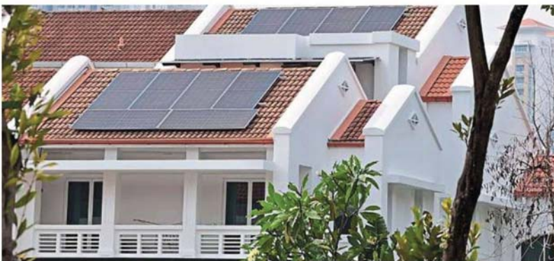
Solar system panel on the rooftop of a residence in Straits Quay, George Town. — ZHAFFARAN NASIB/The Star
