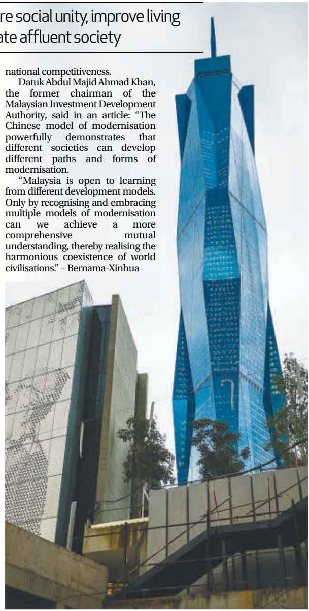
The newly unveiled Merdeka 118 Tower in Kuala Lumpur reflects the nation's march towards prosperity. - BERNAMAPIC
