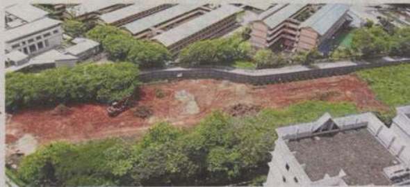
A view of the proposed development site sandwiched by Tiara Faber condominium and SK Taman Desa, along the narrow stretch of Jalan Desa Bakti 2, Taman Desa, Kuala Lumpur.
