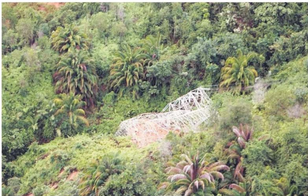
The fallen transmission tower.
