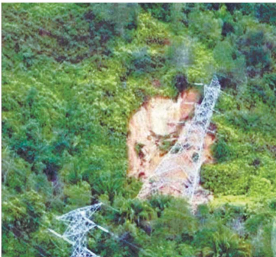
The transmission tower which collapsed following the landslide at Kampung Sarapung.
