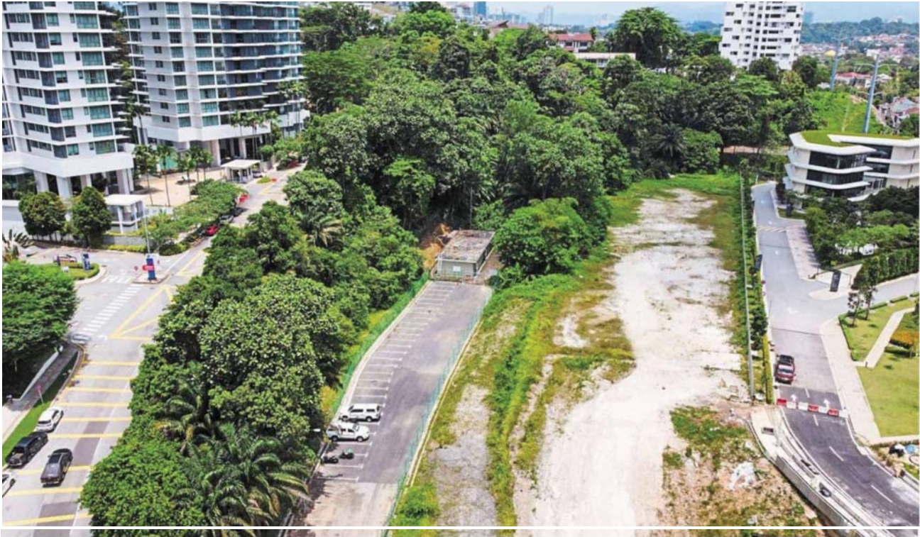
The 2.3ha land for the proposed project in Bangsar, Kuala Lumpur. — Photos: IZZRAFIQ ALIAS/The Star
