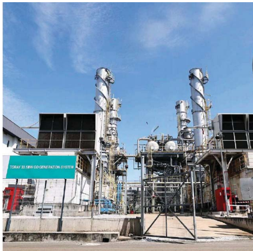
The key benefits of the system are energy efficiency of 75 per cent (versus 45 per cent of the single-generation system) as it also captures heat from electricity generation. — Bernama photo
