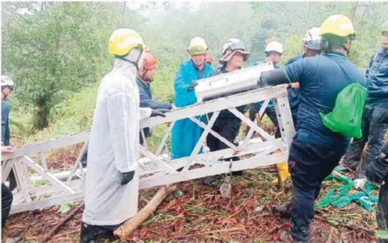
SESB technical team lifting equipment to build the ERS tower.
