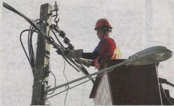
A TNB technician replacing the electric cables and joints in Jalan 17/46, Petaling Jaya.
