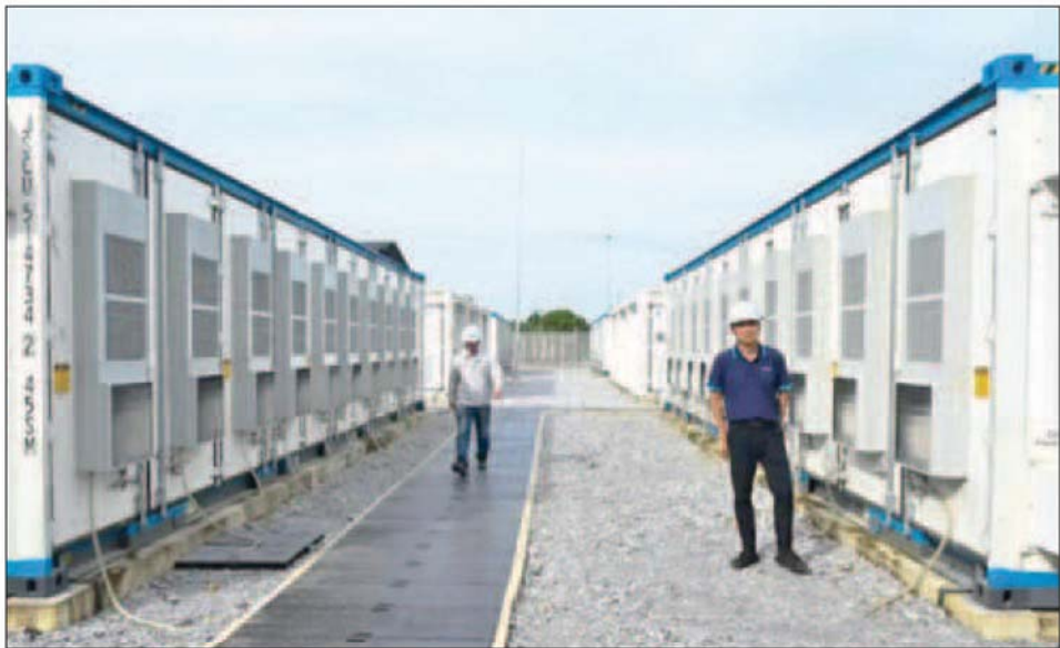
Sarawak's 22-container 60MW battery energy storage system at the Sejingkat power plant.
