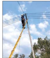
A SESB technician changes the tapping point for one home in the village to a different phase on the transmission lines nearby.
