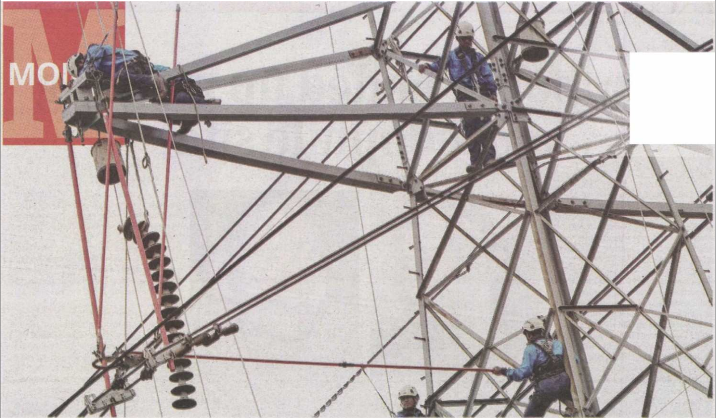
TNB Live Line Unit workers changing porcelain insulation in a 275 kilovolt live line tower near Kapar. — Pictures by Bernama
