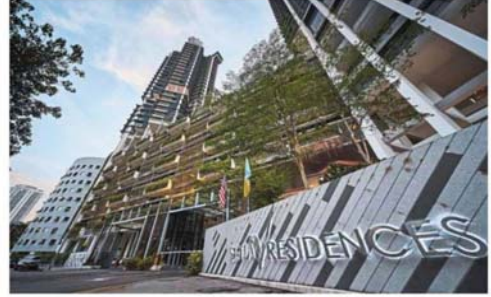
Constructed around a heritage building, Setia V Residences stands as the tallest high-rise residence along Gurney Drive.
