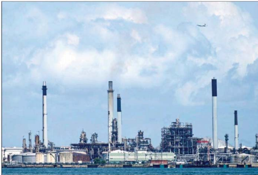
Singapore who is the currently leading DC market in Asia with 53 per cent of the Asean capacity has capped its new data centre builds at 60MW of new capacity per year to
