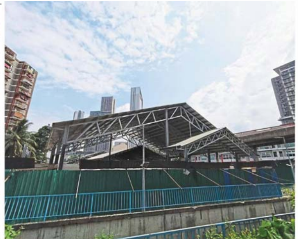
Construction of the new market is now 80% complete.
