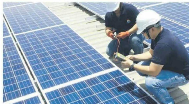
The RM401 million EPCC contract from TNB Kula Muda Solar Sdn Bhd is to develop a 500MWac solar power plant under LSS5 in Bukit Selambau, Kedah, with completion targeted by July 2027.
