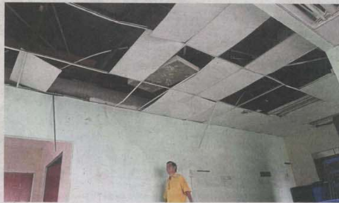
The ceiling of this hall in Bandar Tun Razak is in dire need of repairs.
