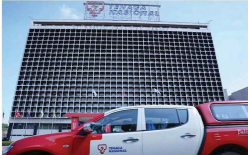
In 2020, TNB together with Malaysian Green Technology and Climate Change Centre (MGTC) have installed 73 EV charging stations in 31 locations.
