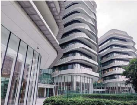
The TNB Platinum Headquarters Campus features high-efficiency building systems and monitoring technologies
