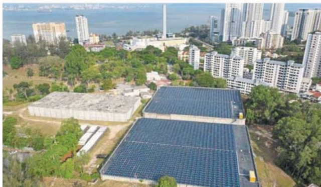
A solar power system at Bukit Dumbar, Penang. In 2021, it generated electricity bill savings averaging RM22,811 a month. – PBA Green Technology
