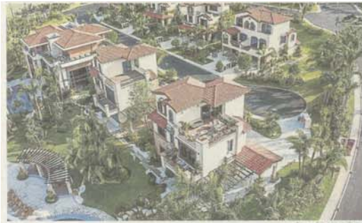
The development by Country Garden Malaysia which was launched in 2014 with some homes equipped with solar panel systems
