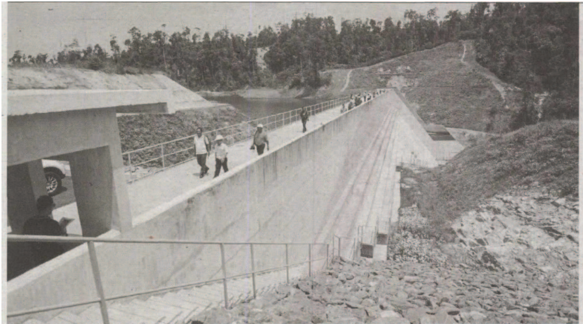
The Tembat dam has been built using German and Swiss technology and is located 429m above sea level. Pic by Mohd Syafiq Ridzuan Ambak
